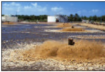
Air-activated sludge lowers the dissolved oxygen content and faecal coliform levels.
