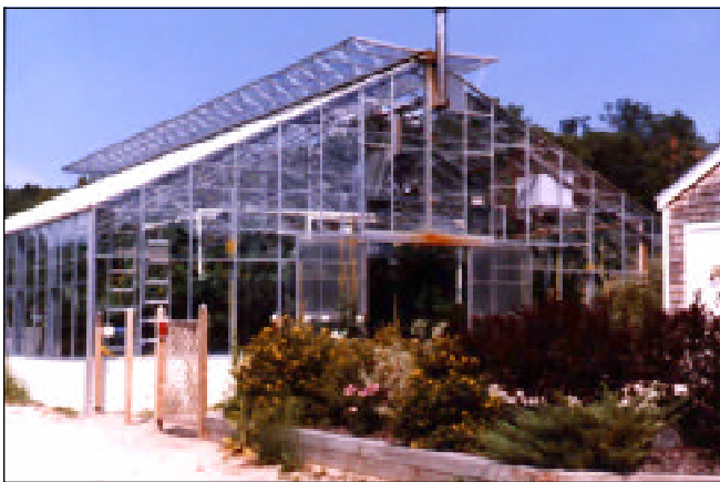
The Bear River solar aquatic sewage treatment facility.
