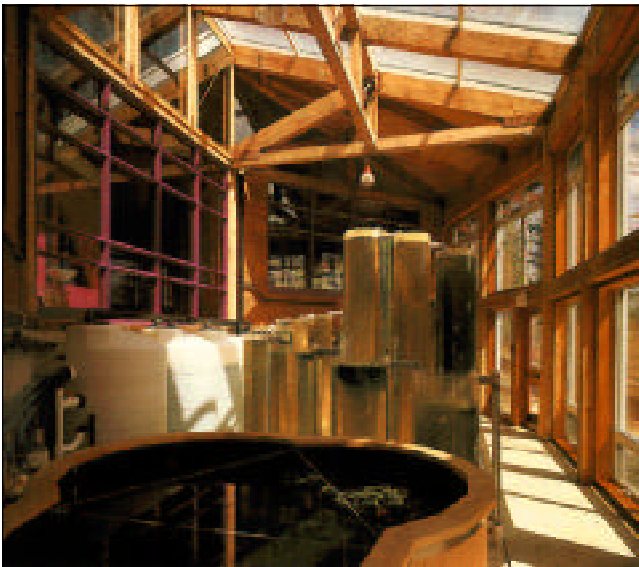
Digestion cells and solar aquatics at the Boyne River Ecology Centre
